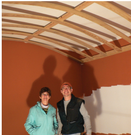
AI President and CEO Mike Wetzel shows his mother, Glenda Wetzel, the ceiling details he hand-built into his new 600-bottle cellar under construction in Skaneateles, New York. A ducted, water-cooled Wine Guardian with humidifier is installed in an adjacent mechanical room and mounted over the entrance door to conserve space.
